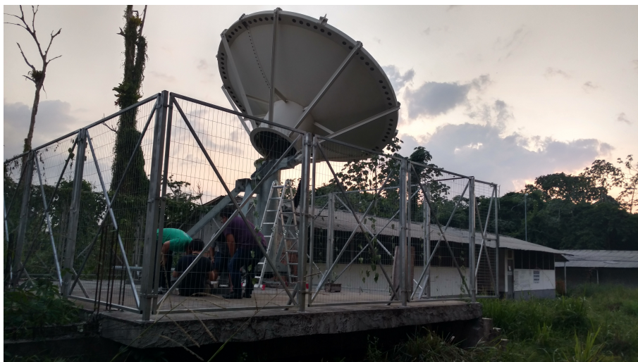
Figure 2.3: 3 axes antenna installed at PCT Guamá.
