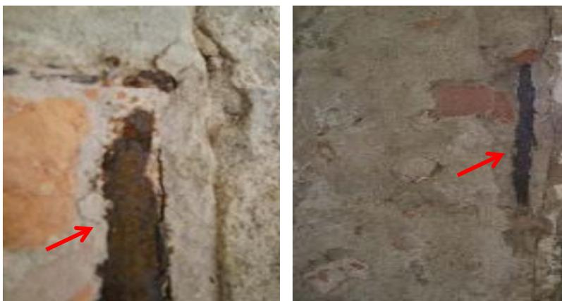
Figura 4.6 – Vista do pilar com armadura de  $\varnothing 10,0$  mm (SEOP – AC)
