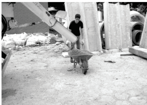
Figure 9 – Concrete placement and slabs' surface regularization
