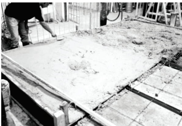
Figure 9 – Concrete placement and slabs' surface regularization
