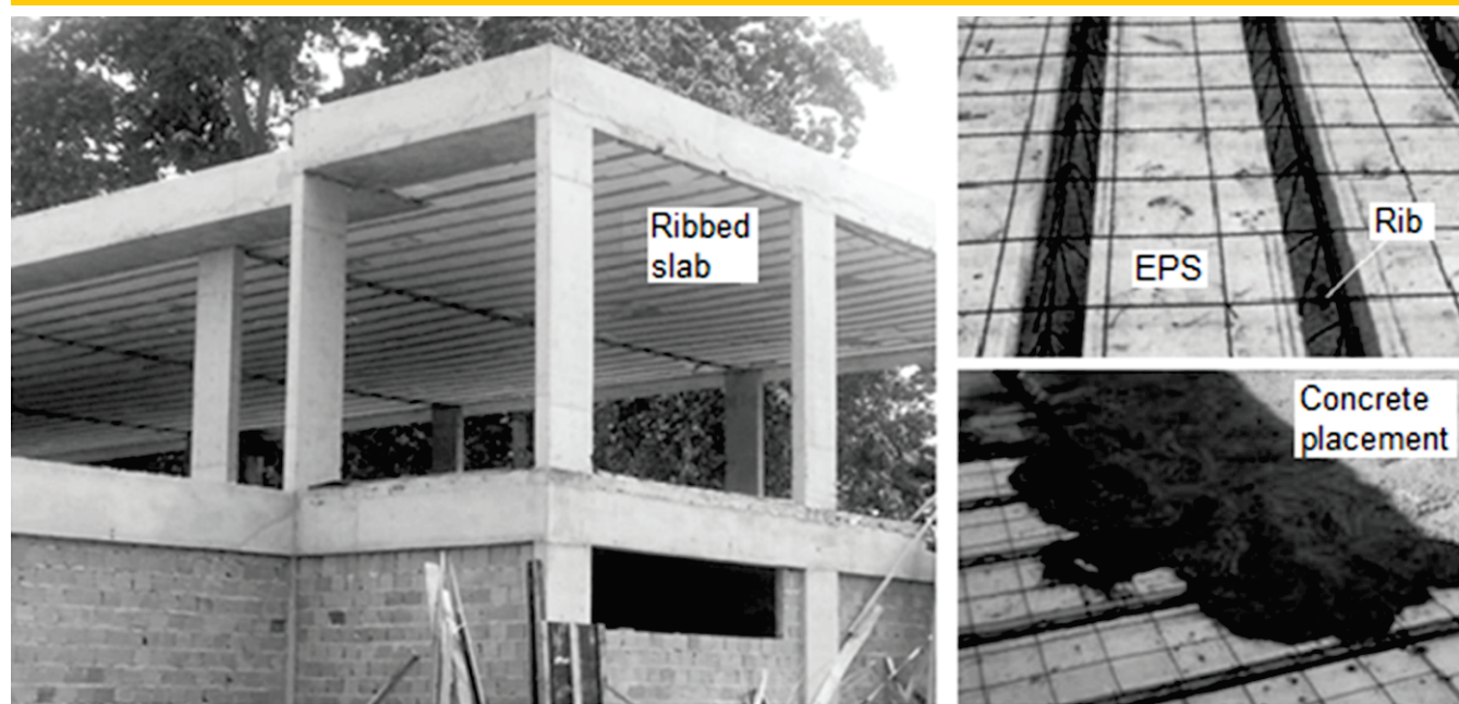
Figure 1 – One-way ribbed slab
