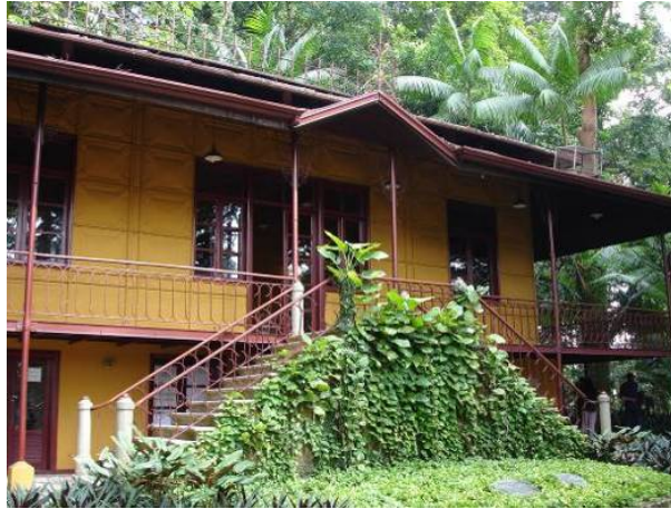
Figure 02 - Iron chalet at Rodrigues Alves Botanical Garden.
