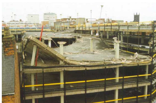
Figura 1.4 – Prédio Pipers Row Car Park, Wolverhampton, Reino Unido (WOOD, 1997)
