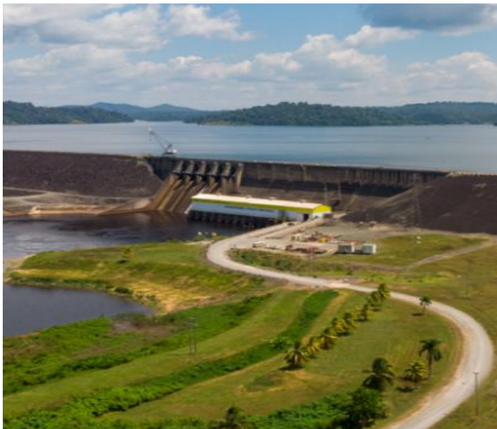
Figura 7 – Afobakka Dam (Brokopondo Reservoir)
