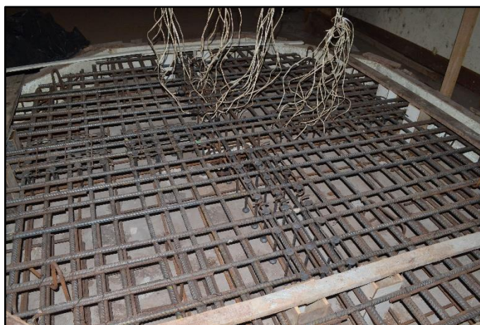
Figura 3.8 – Laje com Double Headed Studs (Autora, 2023).
