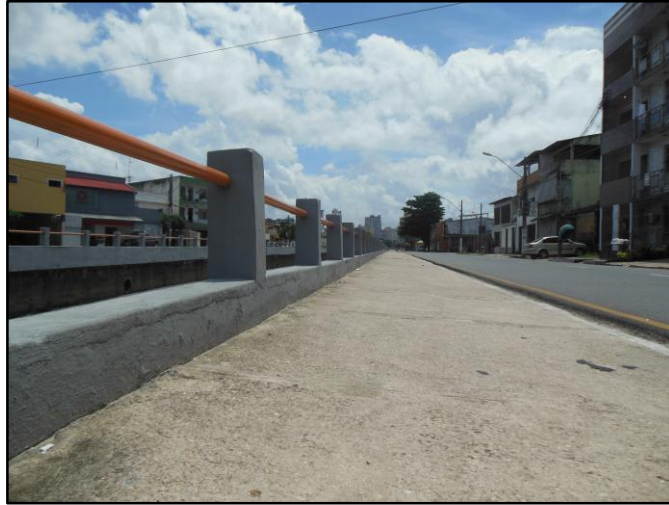
Picture 2 - Poor vegetation in DABEL, 2013. Tamandaré Avenue in Cidade Velha neighborhood.
