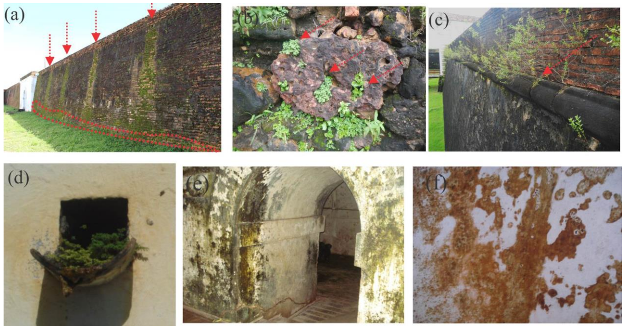
Fig. 8. Bioreceptivity in FSJM: (a) lichens and mosses in bricks of internal scarp in humid areas towards drainage and bottom near the ground; (b) nodular lateritic crust with rough surface favoring the vegetation development; (c) sparse vegetation in west curtain, but concentrated in the raised area of the cord line and in the grooved parapet cracks; (d) ceramic roof toe of internal drainage of vaults bunkers with green algae biofilm and vegetation ( Pilea microphylla ); (e) green and black biofilms in humid areas in South bunker cells; (f) reddish orange biofilm on dungeon walls.
