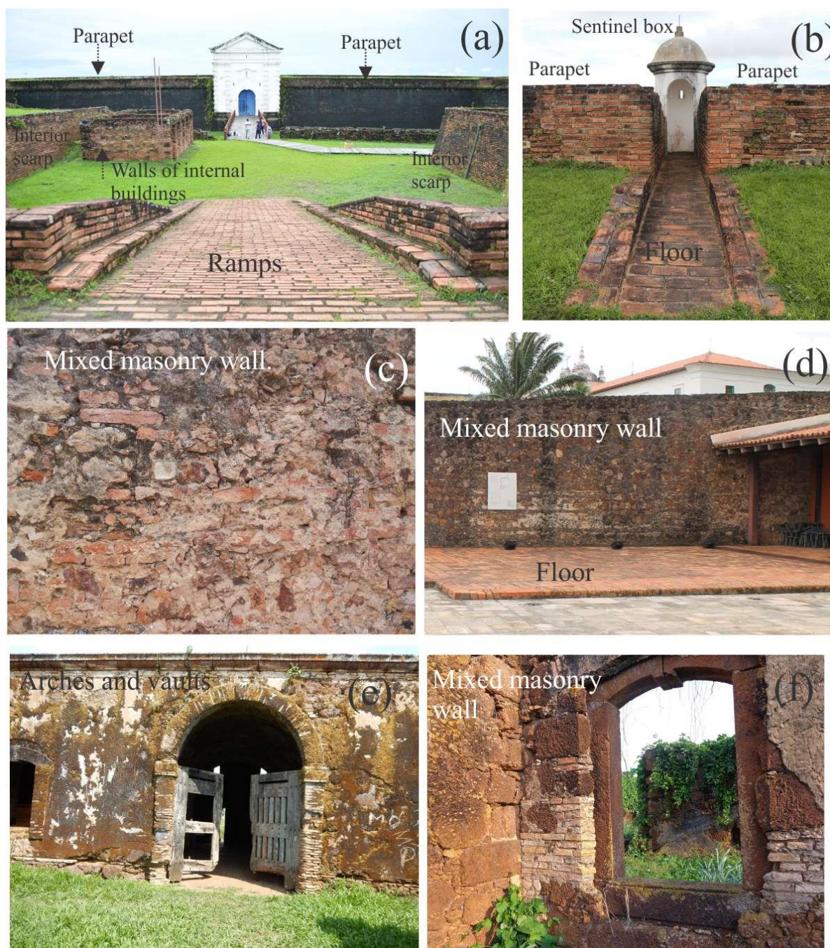
Fig. 26. Different applications of ceramic bricks in the Amazon fortresses: (a, b) HCB and RCB in profusion of use and functions in the FSJM (Amapá); (c, d) HCB in mixed masonry walls and RCB in pavements in the FCPB (Pará); (e, f) HCB in the composition of arches and filling of predominantly stone masonry parts in the RFPB (Rondônia).
