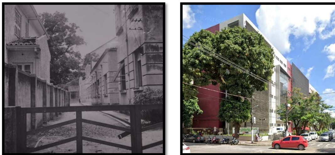
Figura 65 – Lateral do Instituto Ophir Loyola, déc. 1950 e Hospital Ophir Loyola, 2023
