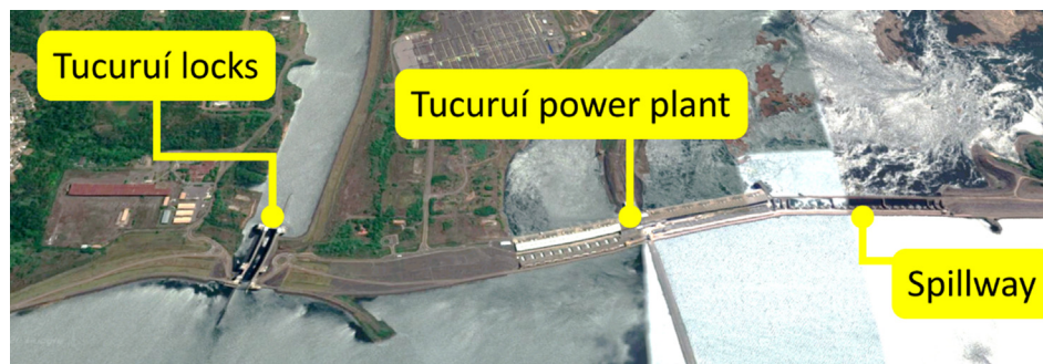
Fig. 1. Overview of the Tucuruí hydropower dam and its locks.
