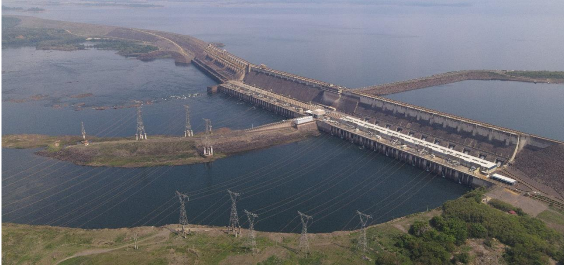
Figure 13 – Tucuruí Hydropower Plant on the Tocantins River.
