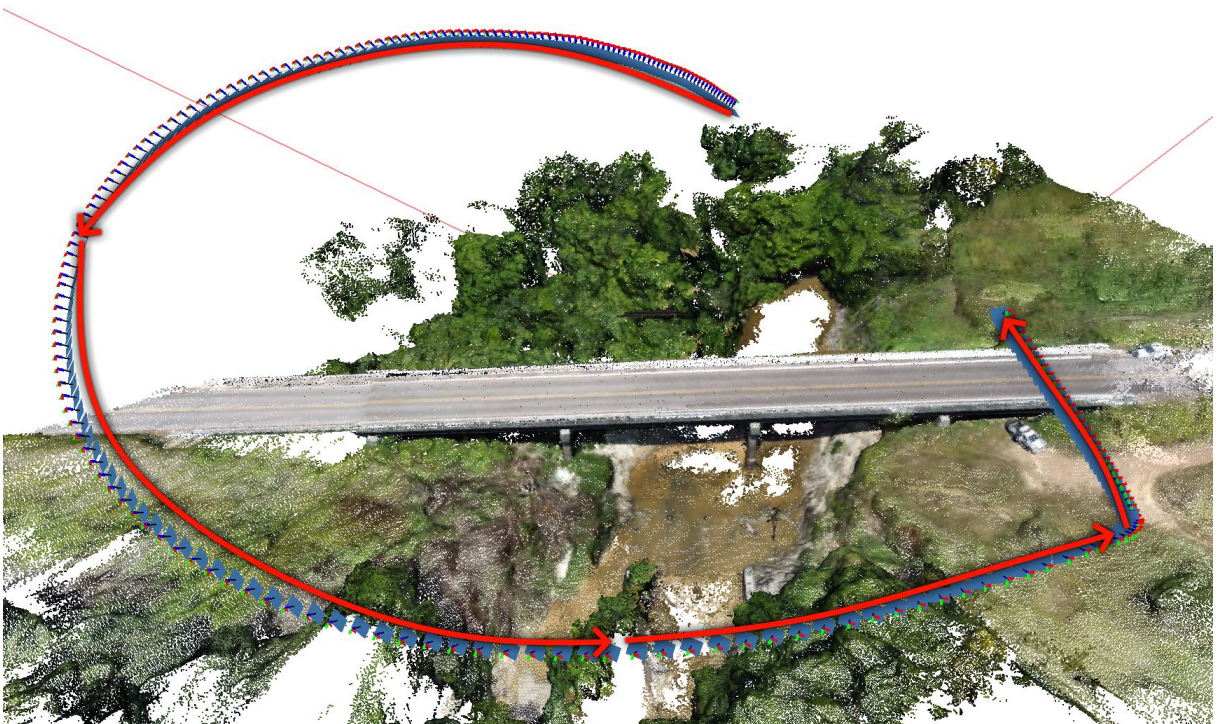
Figure 15 – Camera angles of the photos taken by the drone over the Taurarizinho River Bridge.
