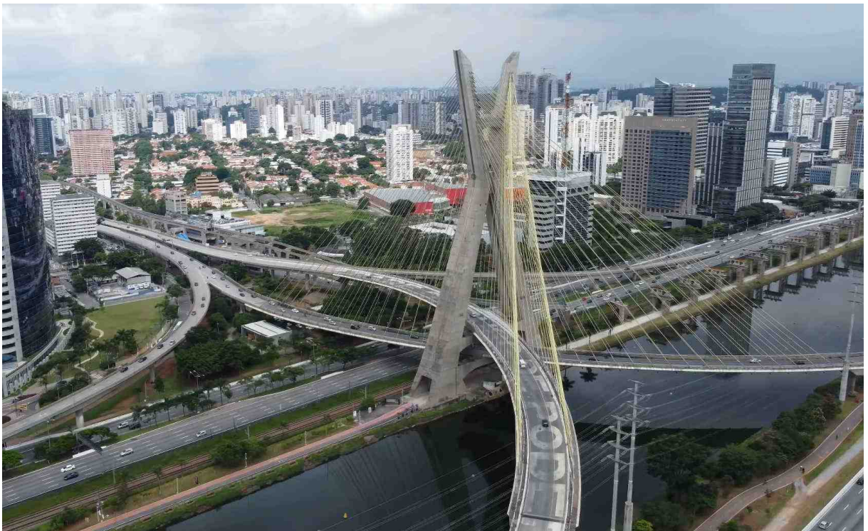
Figure 18 – The Octavio Frias de Oliveira Cable-stayed Bridge crossing the Pinheiros River
