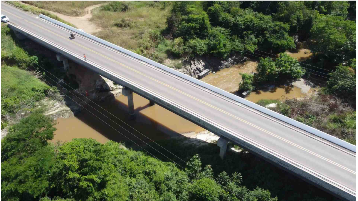
Figure 14 – Side view of the Taurarizinho river bridge
