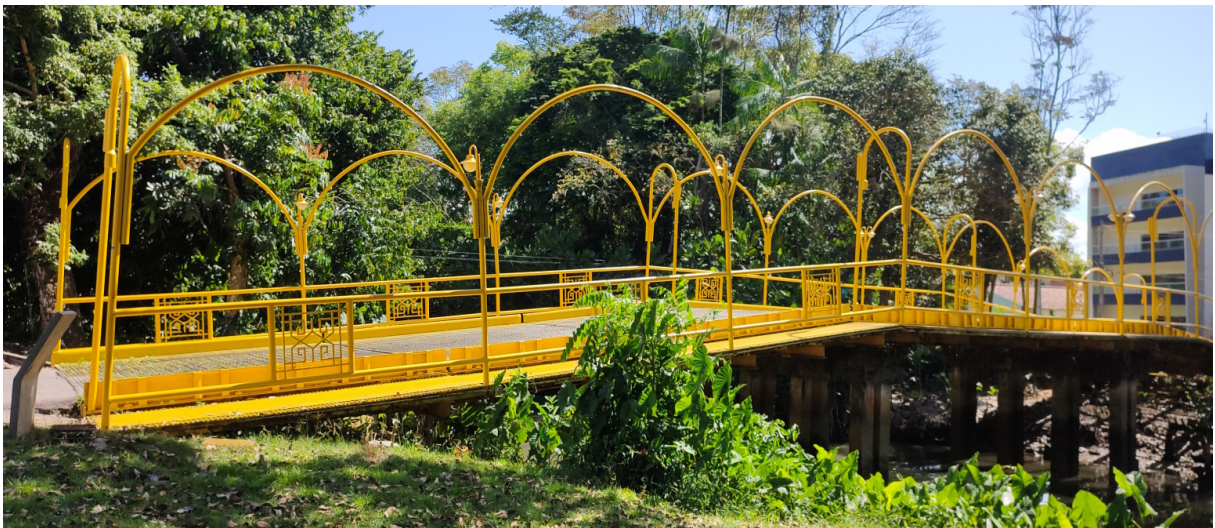
Figure 12 – Side view of the Tucunduba river bridge in the UFPA campus
