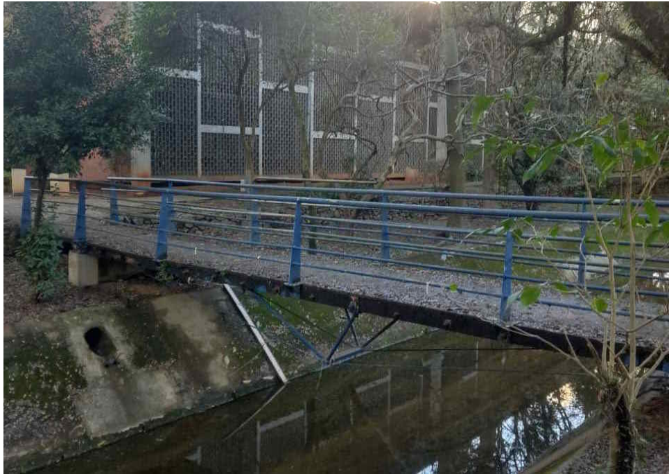
Figure 16 – The USP Bridge over the Tejo stream, São Paulo, Brazil
