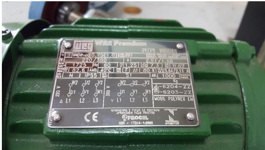
Figure 0-3 – IE3 Class induction motor nameplate.
